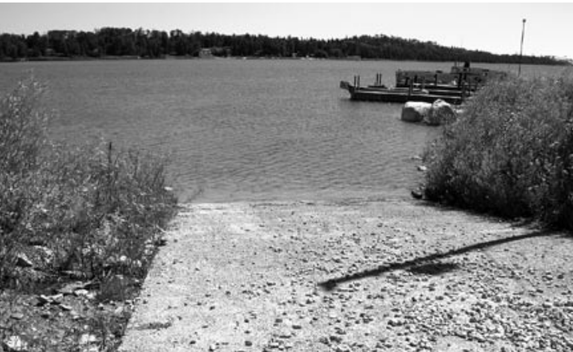
The site was dredged to a depth of 4 feet below low water and boulders moved from the launch site's path.
