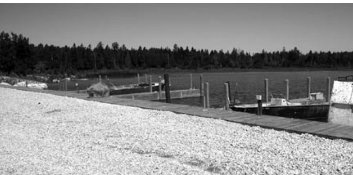
Dredged materials were hauled out and the pier laid with fresh gravel while the 40-foot finger piers were reinstalled.
