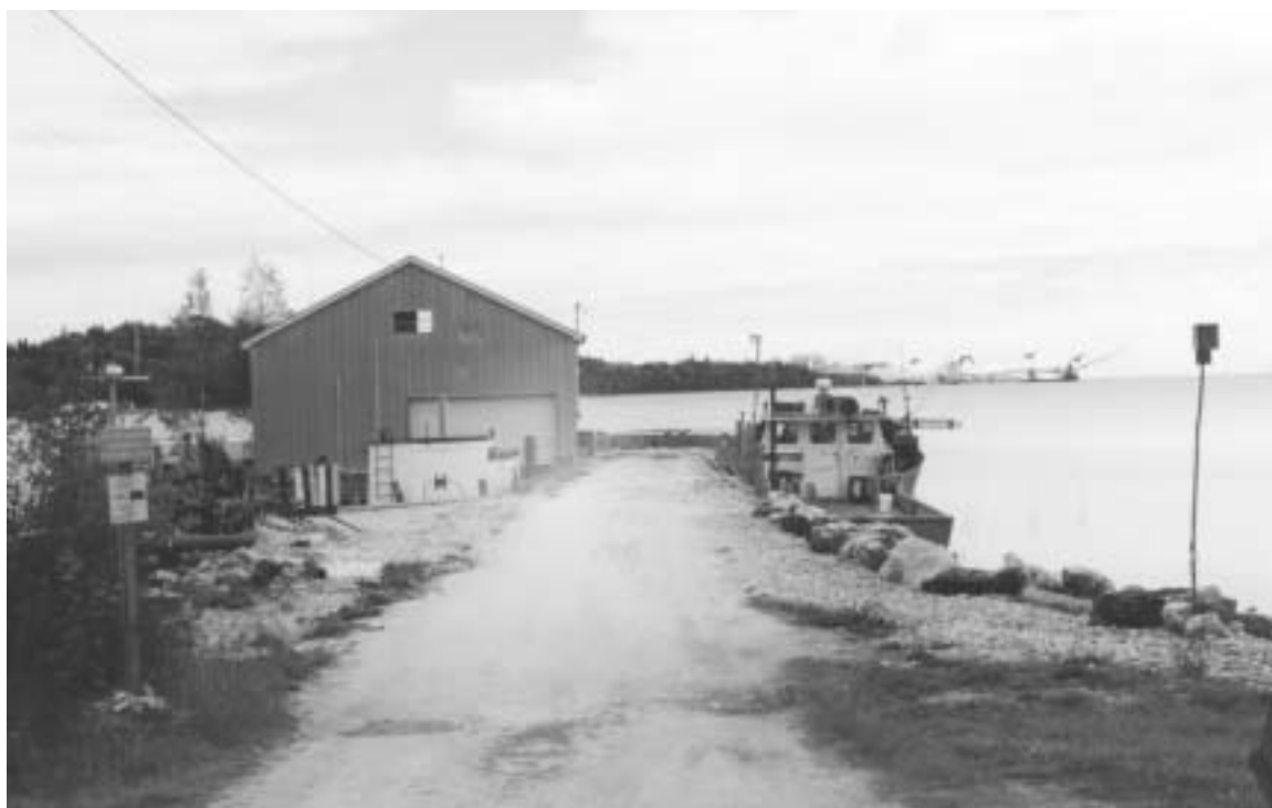
Dutcher's at McKay Bay prior to building removal.
